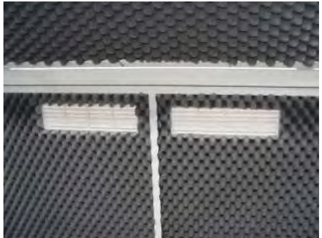
Sound proofing inside walls
